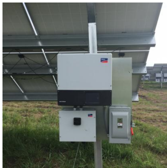
SMA String Inverter/Combiner Box and AC Shutoff
