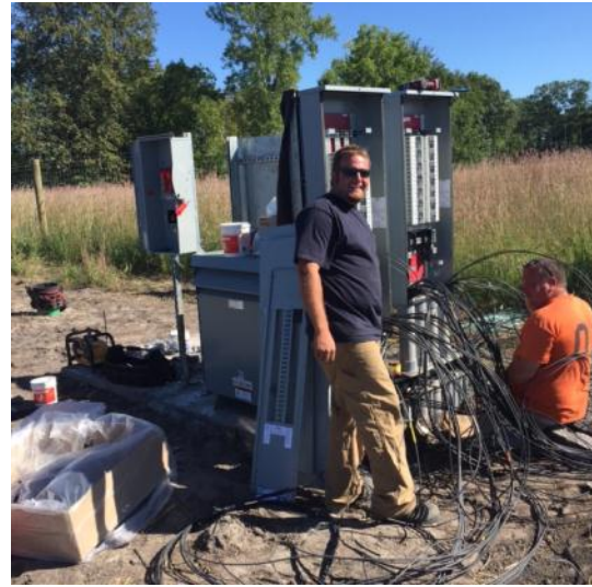
Crews wiring the AC Panels
